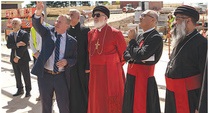
His Holiness Mar Awa III toured the Mar Meelis Zaia AM Sport and Performing Arts Centre while it was still under construction during his visit to the College.
